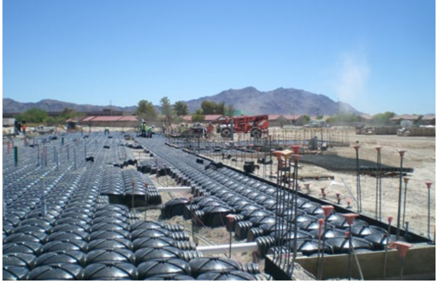
Figure 1 Cupoplex aerated floor void space system. Source: ITRC PVI-1 Guidance Document, used with permission.
