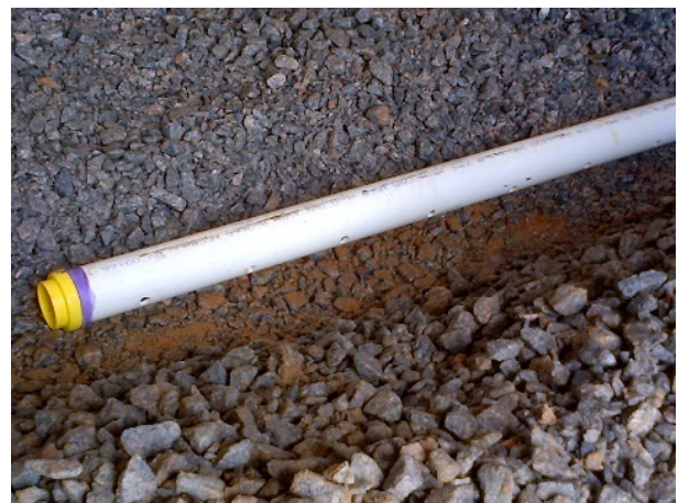
Figure 4. Photograph of mitigation system piping. Source: A. Rodak, Duncklee & Dunham, used with permission.
