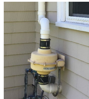
Figure 3. Blower installation outside building.
