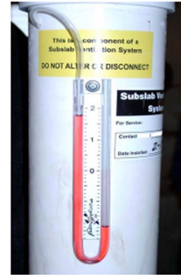
Figure 5. Typical U-tube manometer.
