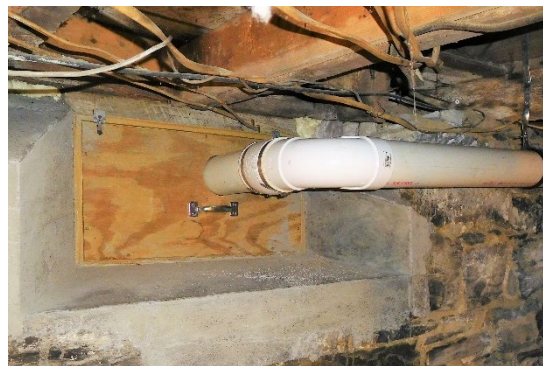
Figure 2. Example piping into a crawlspace area. Source: C. Regan, ERM, used with permission.
