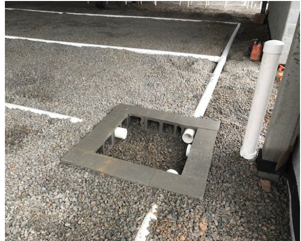
Figure 5. Photograph of a header for mitigation system piping. Source: Dunclee & Dunham, used with permission.
