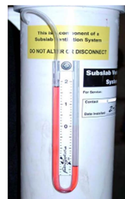
Figure 5. Typical U-tube manometer.
