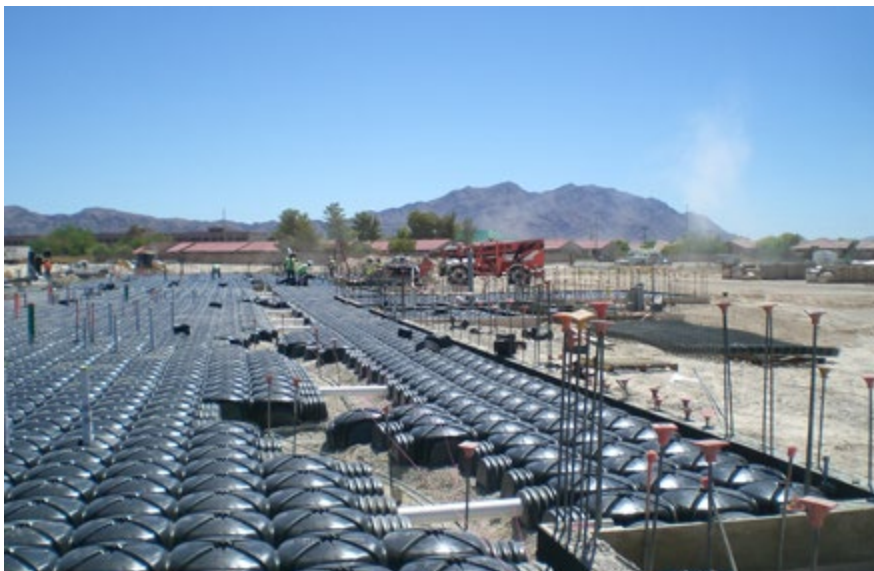
Figure 1 Cupolex aerated floor void space system. Source: Vapor Mitigation Sciences, LLC, used with permission.
