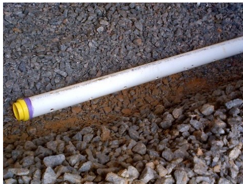
Figure 4. Photograph of mitigation system piping.
