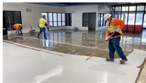
Figure 1. Application of EFC to a concrete substrate.
