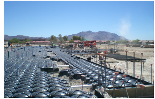
Figure 1 Cupolex aerated floor void space system. Source: ITRC PVI-1 Guidance Document, used with permission.
